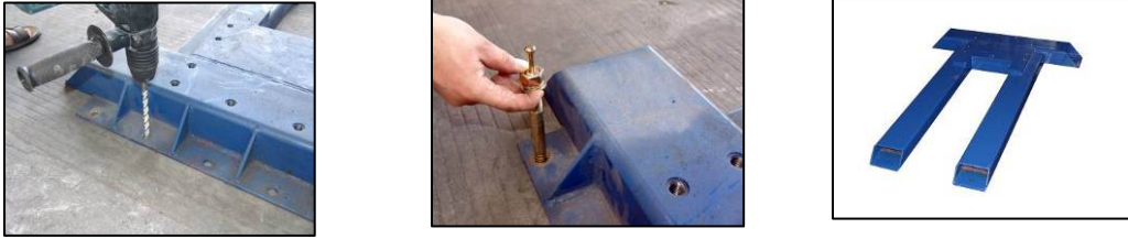
Fig. 3- A, B, C Anchoring the base plate
